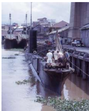
HMS Tabard damaged after being swept into Howard Smith Wharf by a strong current, March 29, 1963.
